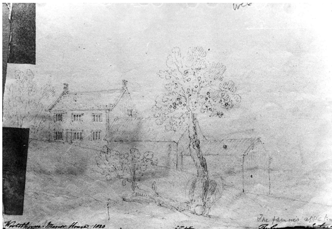
Figure 3. Newton's apple tree in the garden of Woolsthorpe Manor, drawn by the Rev. Charles Turnor in 1820. The 'fan shaped' protrusion represents the broken trunk of the tree which can be seen in figure 4. (Private collection.)
